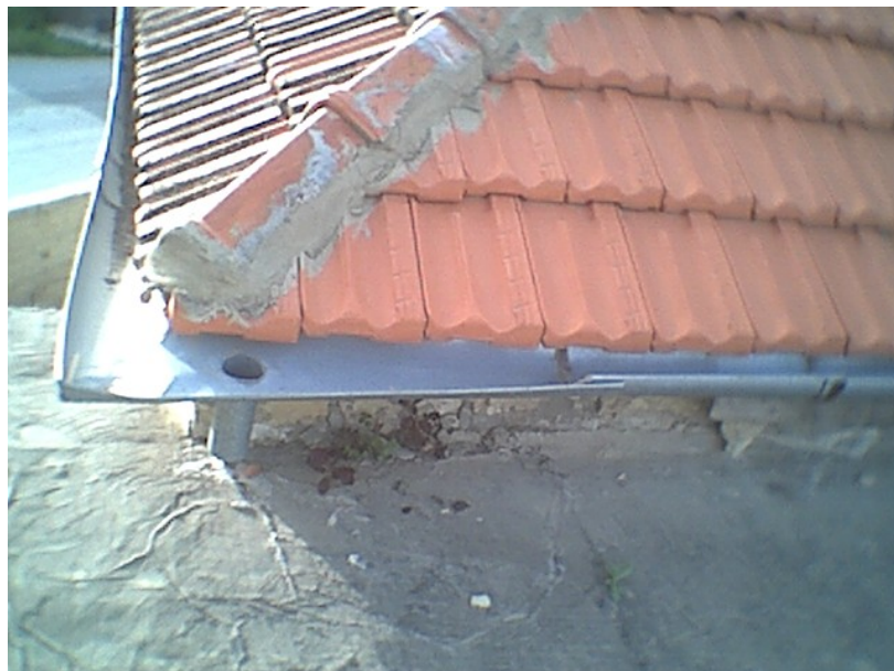
Photo 3.5.1: Galvanized steel gutters (Ramallah).
