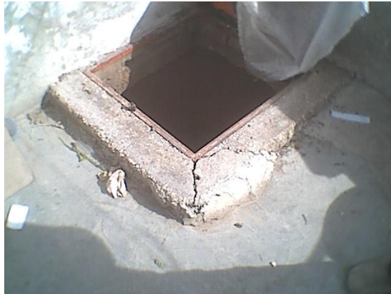
Photo 3.7.1.4: Contamination due to poor maintenance (Abu Shekheidim).
