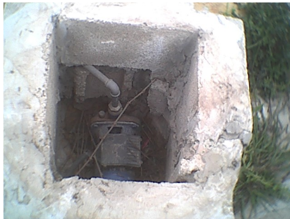
Photo 3.5.4: Delivery system by using pumps (Kubar).
