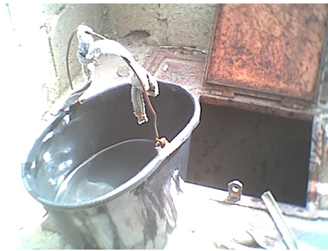
Photo 3.7.1.2: Contamination due to collecting water directly in bucket (Kubar).
