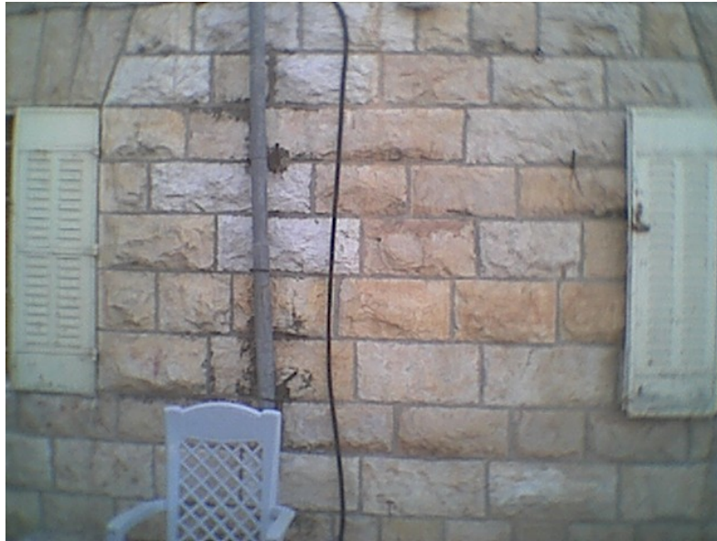
Photo 3.5.2: Galvanized steel downspout (Abu Shekheidim).
