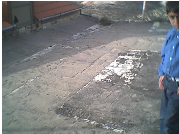
Photo 3.7.1.1: Contamination due to dirty catchments surface (Abu Shekheidim).
